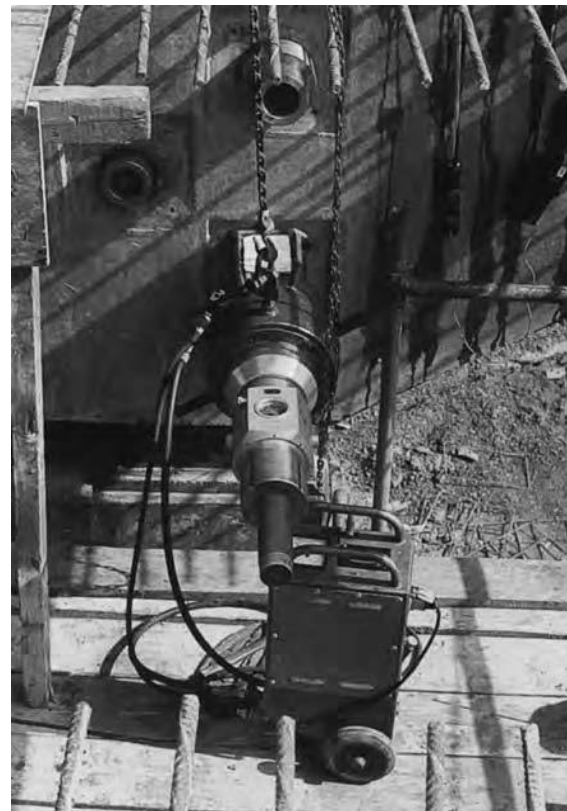
Figure 11.9 – Typical Hydraulic Jack (with hydraulic hoses from compressor unit foreground)
