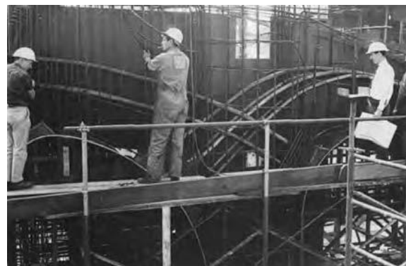
Figure 11.8 – Positioning the Ducts in the Formwork
