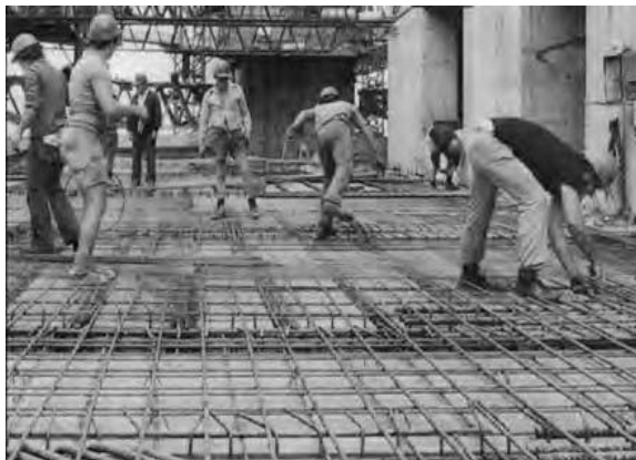
Figure 11.2 – Reinforcement being tied in Position
