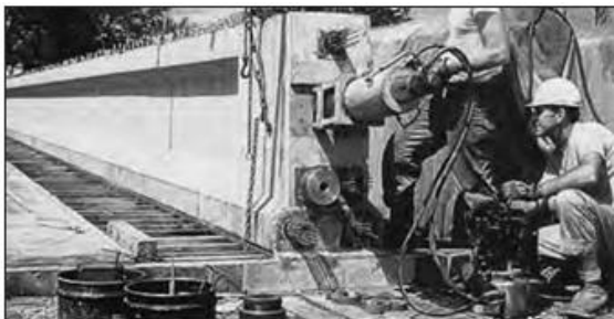
Figure 11.6 – Post-tensioning Jack operating on End of Concrete Girder
