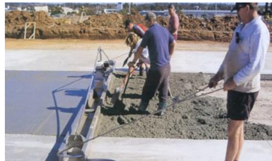
Figure 13.7 – Typical Vibrating Screed Surface Vibrator
