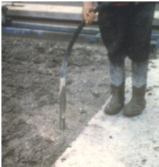
Figure 13.9 – Use of an Immersion Vibrator at a Slab Edge
