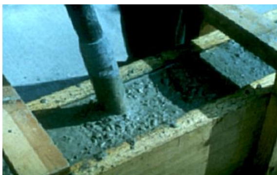
Figure 13.3 – Using an Immersion Vibrator
